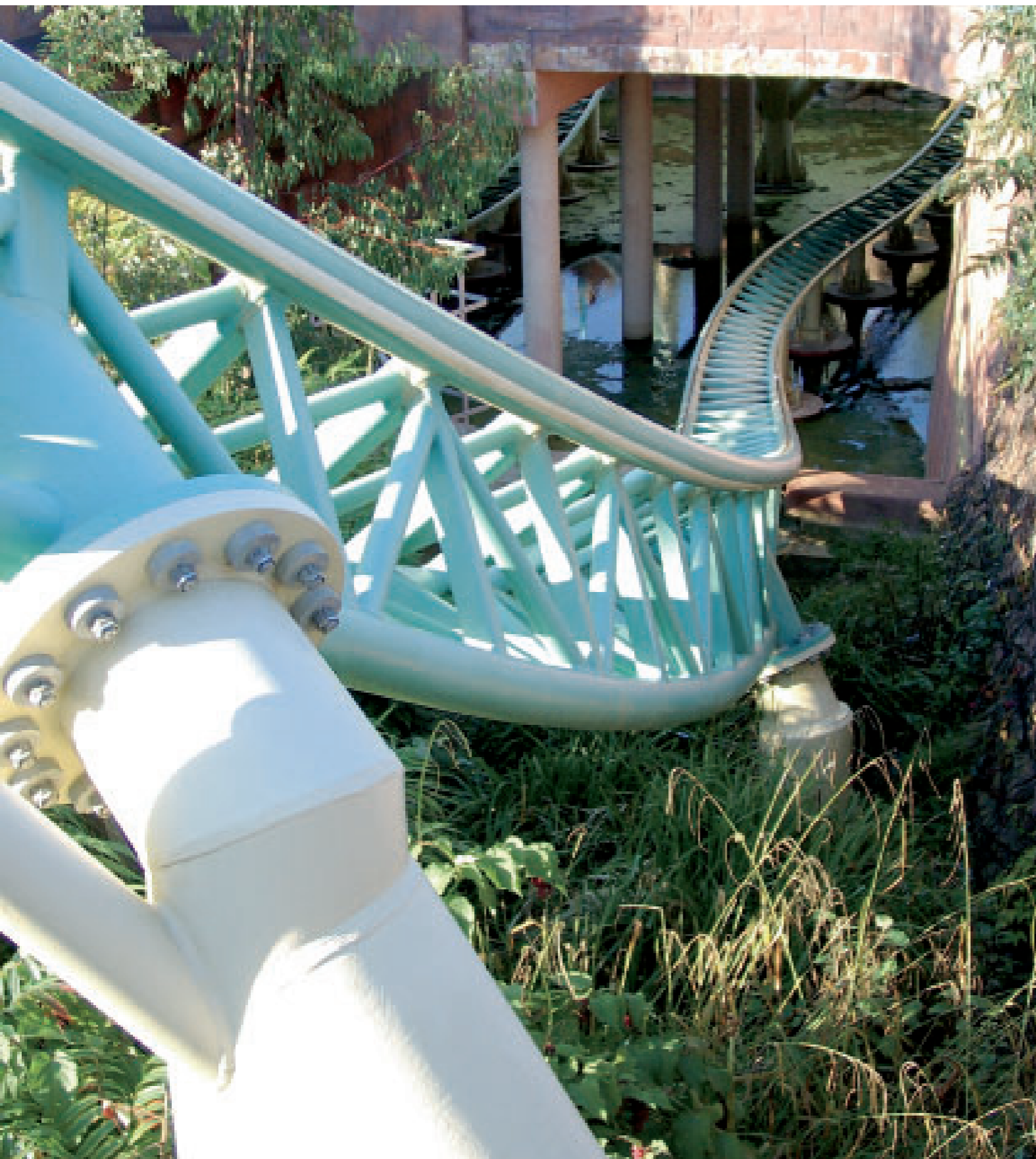
Steel can stand it: Supports for a spiral roller coaster.
